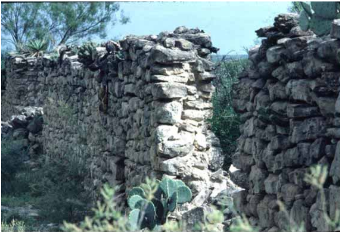
Figure 6. Standing walls at Monclova Viejo (courtesy of John Stockley).
